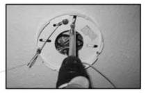
(3) Secure suspension cable loop around the hook inside the top of the fan body.
