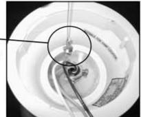
(4) Lift fan body and carefully align collar with ceiling plate. Tabs on ceiling plate should seat into channel on inside of fan collar. Rotate fan so that set screw holes on fan body align with set screw holes on ceiling plate.
