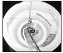
(4) Lift fan body and carefully align collar with ceiling plate. Tabs on ceiling plate should seat into channel on inside of fan collar. Rotate fan so that set screw holes on fan body align with set screw holes on ceiling plate.
