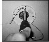
(3) Secure suspension cable loop around the hook inside the top of the fan body.
