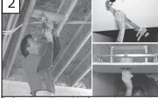
Before installing this fan make sure the outlet box is properly installed to the house structure. To reduce the risk of fire, electric shock, or personal injury, mount to outlet box or supporting system acceptable for fan support.
