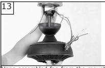
Hang assembled fan from the mounting bracket installed to ceiling in previous step. Make sure the fan is hanging straight. Rotate fan until the tab on the Mounting bracket engages the slot on the Downrod Ball. This must be done to prevent the fan body from rotating when the blades are in motion.
